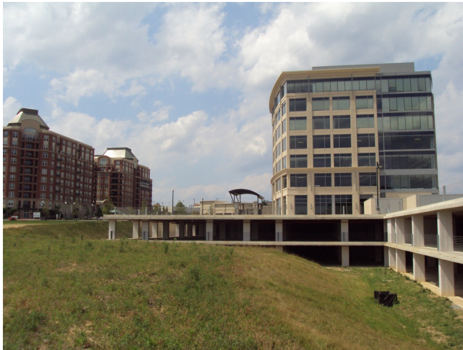
Figure 6: View from North
