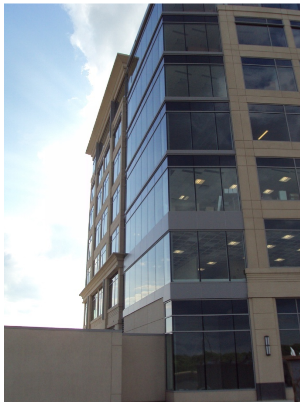
Figure 12: Slab End Cantilever Provides Seamless Glass Corners
