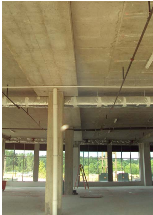
Figure 13: Shallow, Wide PT Beams
