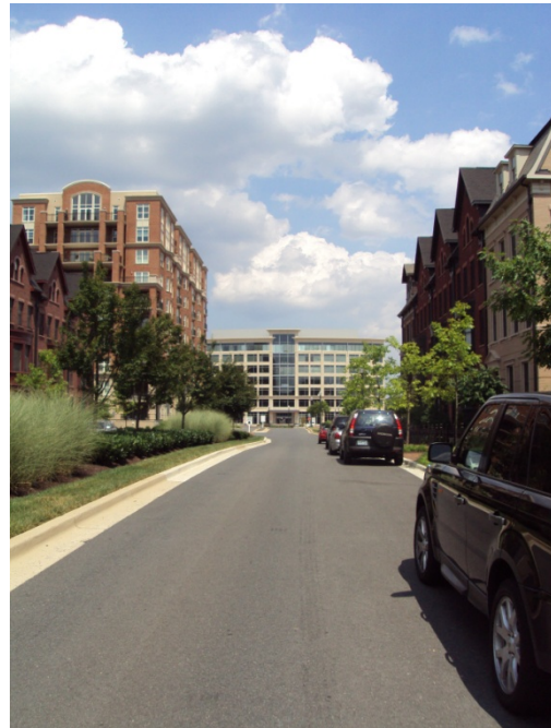
Figure 1: View from Cadbury Ave.
